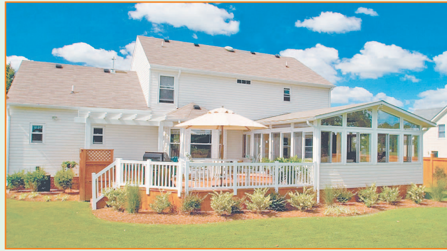
This sunroom and deck with pergola over a hot tub area are among the many successful projects that Outdoor Designers has undertaken to help clients enjoy their outdoor spaces.
